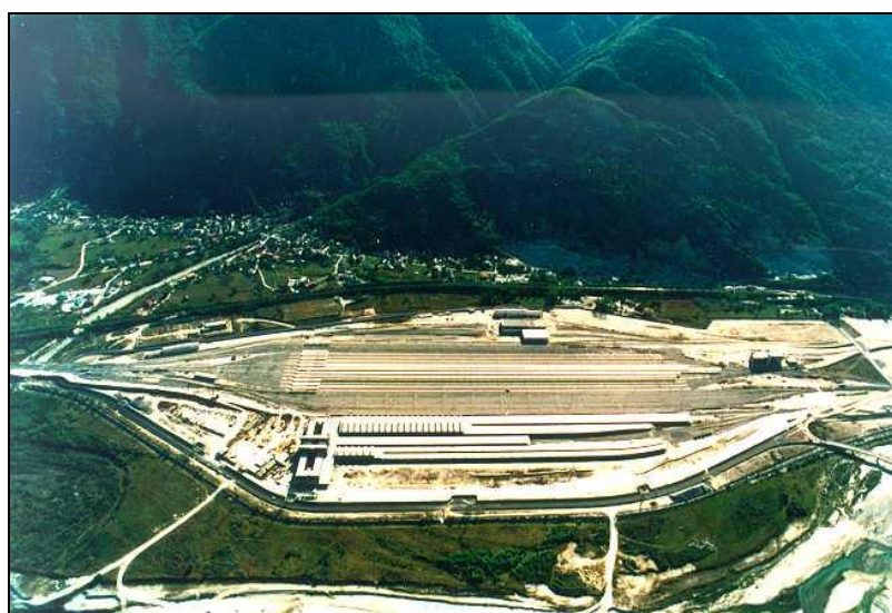
International Goods Station of Domodossola (Italy/Switzerland)
