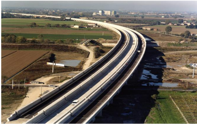
High Capacity railway line Milano-Bologna
