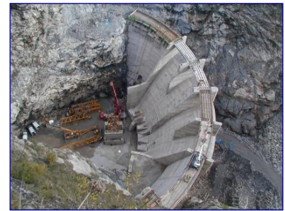
Gorge di Susa Dam (Alps)
